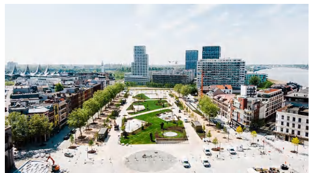
Figure 1: Antwerp Zuiderdokken - cars underground
