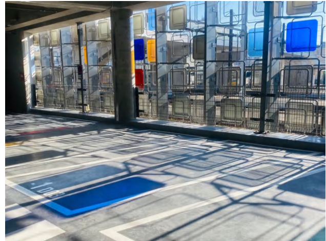
Figure 22: Q-Park Gare Colisée - coloured glass façade
